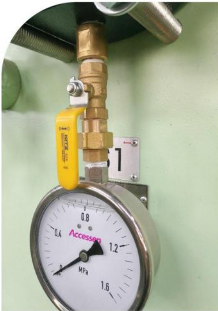
Marine liquid filled pressure gauge
